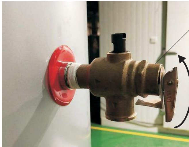
Figure 4: Air removing process
